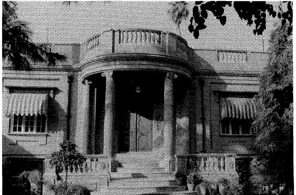
After World War I, local craftsmen implemented designs from the West in collaboration with, and under the supervision of, Iraqi civil engineers
