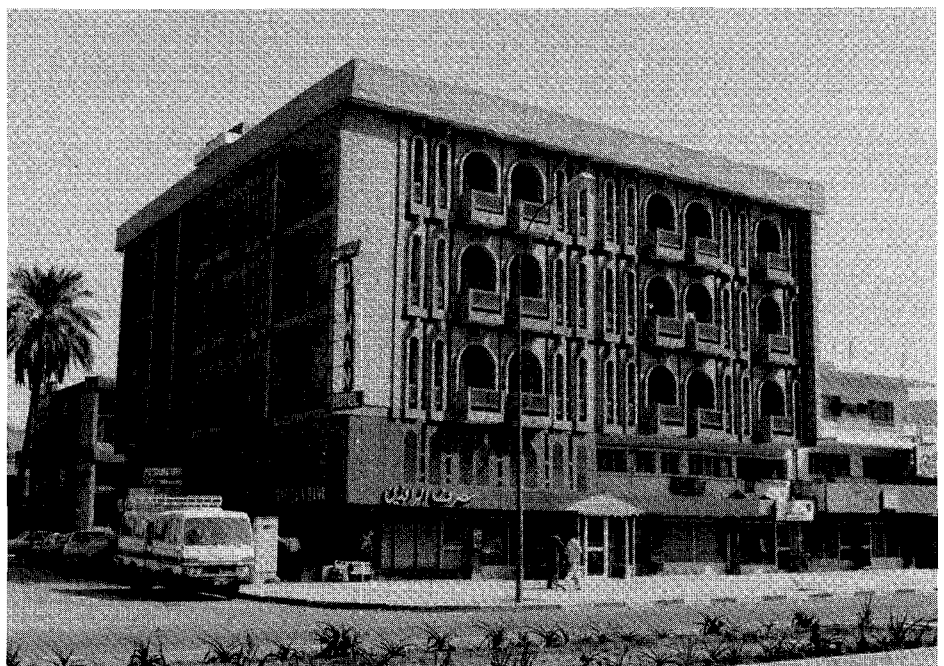
Baghdad, a structure typical of the late 1970s.
